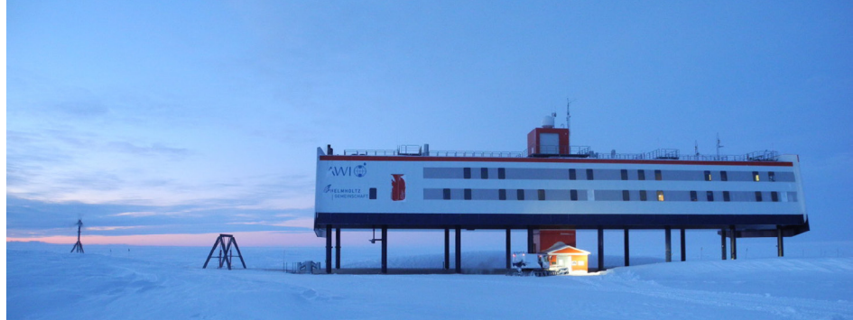
Photo 1: The German Antarctic Research Station Neumayer III at the Ekström Shelf Ice in the north-eastern Weddell Sea (70°40'S, 08°16'W) started routine operation in 2009. The building is situated on a platform above the snow surface integrating scientific research (meteorology, air chemistry and geophysics), operational and accommodation facilities in one building, and it is connected to a garage in the snow. The red hall located at the center of the roof is the platform for launching weather balloons. The picture was taken during polar night in June 2012. © Kathrin Höppner.
